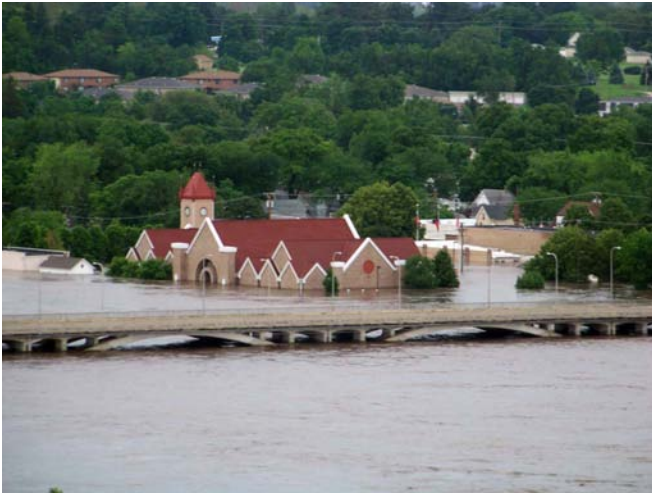
Czech & Slovak Museum submerged in flood waters just under 12 feet deep. June 12, 2008, prior to crest.
