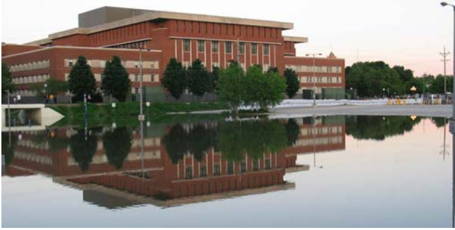
Flooding on west side of UI Libraries, June 13, 2008. Prior to river crest.
